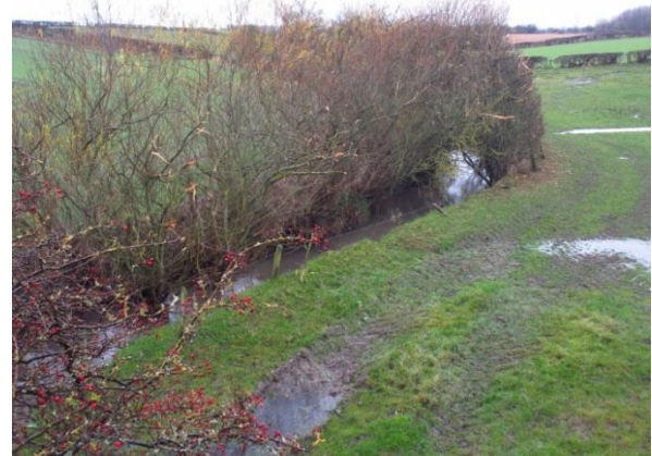
Figure 3.2: Eroding bank exacerbated by poaching
